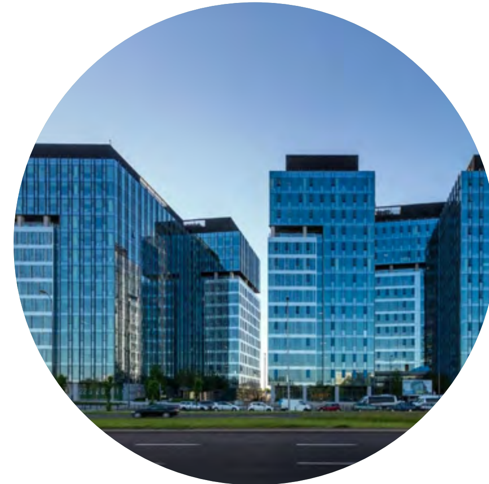
Warszawa, West Station I-II, 144 000 mkw., 2020-2022
