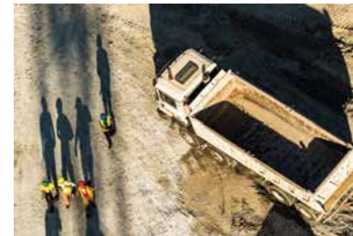
Up to the beginning of this year we have removed approximately 200,000 m 3 soil from the construction site, transported daily by an average of 45 trucks, preparing the area for the structure building works.
