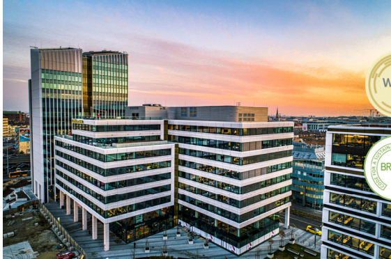
Agora Tower & Hub, Budapest
